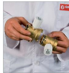
to lightly lubricate the O-ring with silicone grease if necessary. To prevent any material from entering and damaging the O-rings, it is a good idea to wait until the moment of assembly before taking the modules out of their packaging. To enable the bayonet connection of the individual modules, position them side by side with their vertical axes rotated by 90°.
