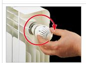
**3)** Fully close the head by turning the knob (turn the knob to position \*).
